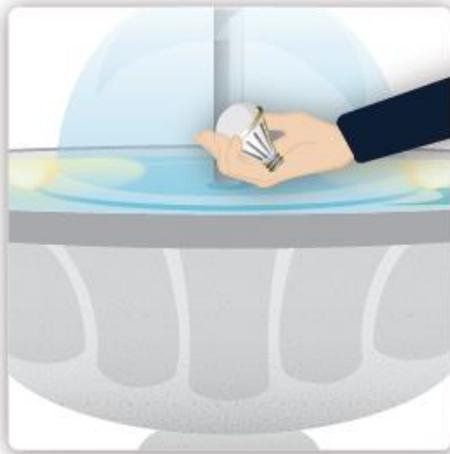
3. Anson decides to replace the incandescent bulbs with LED bulbs to prevent the lights from heating the water to a temperature that allows biofilm to grow.
